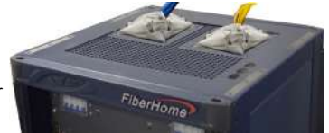
Fastening the mouseproof hop-pockets on the top of the cabinet
